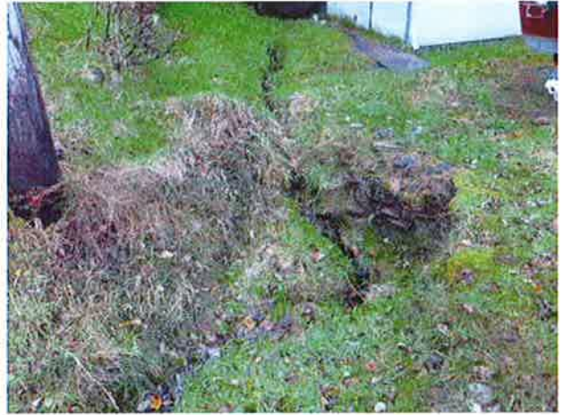
Incised channel from seep or foundation drain on property leading to inlet.
