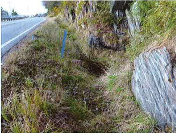
Inlet and ditches to north.
