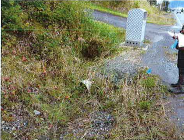
Aluminum extension of inlet, mailbox, and ditches to south.
