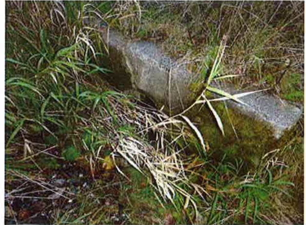
Concrete headwall at inlet.
