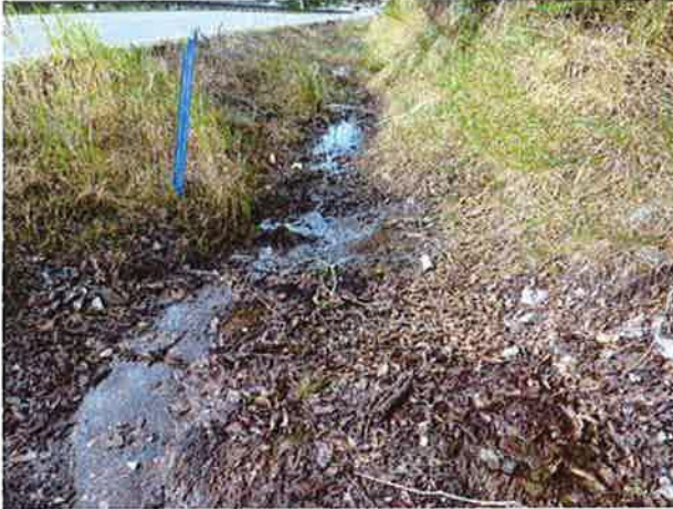
Inlet at blue marker, ditches to north.
