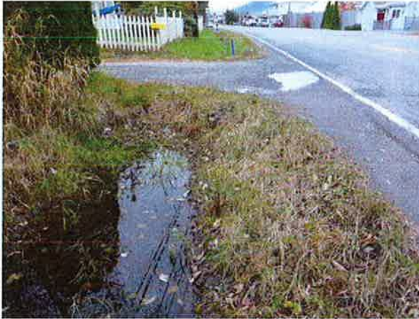
Ponding water in ditch north of inlet; views looking south toward inlet marked by blue post.
