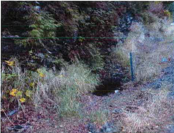
Inlet and ditches to south.
