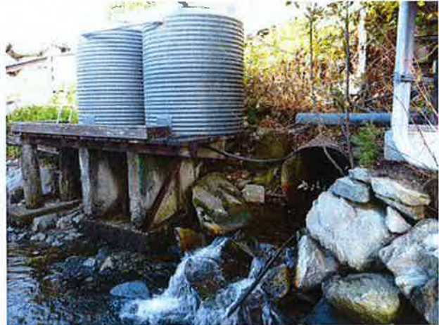
Surrounding structures at outlet.
