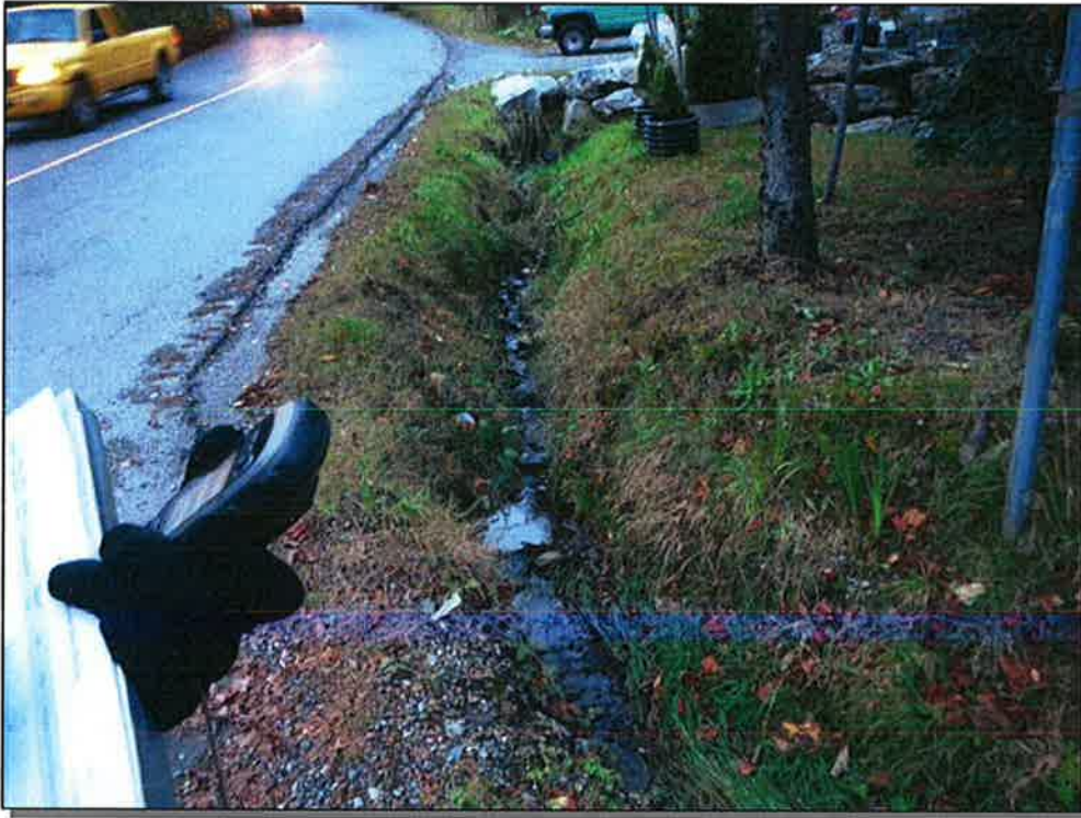
Site 017: Stream Crossing, Upstream View. Photo taken October 14, 2015.
