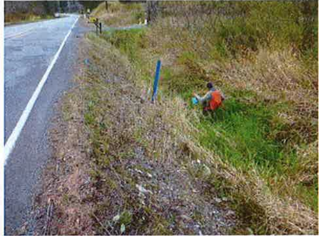
Inlet and ditches to north.
