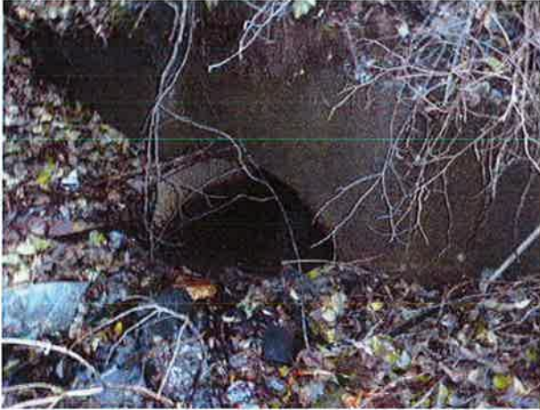
Inlet with concrete headwall.
