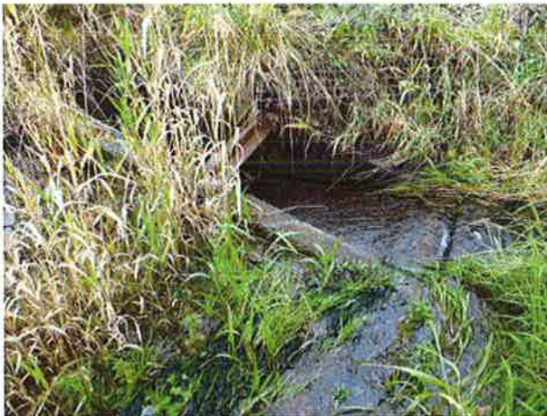
Inlet to south draining marsh area.
