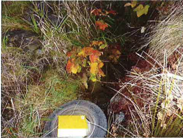
Inlet in heavily vegetated area.
