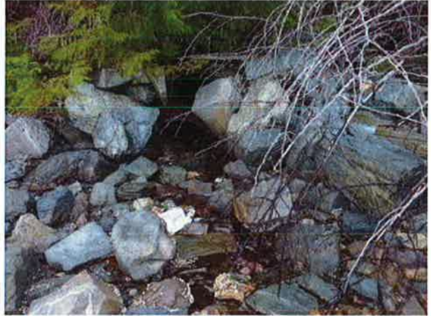
Outlet corroded and damaged.
