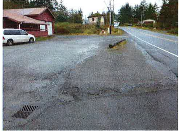
Another curb inlet, looking south.
