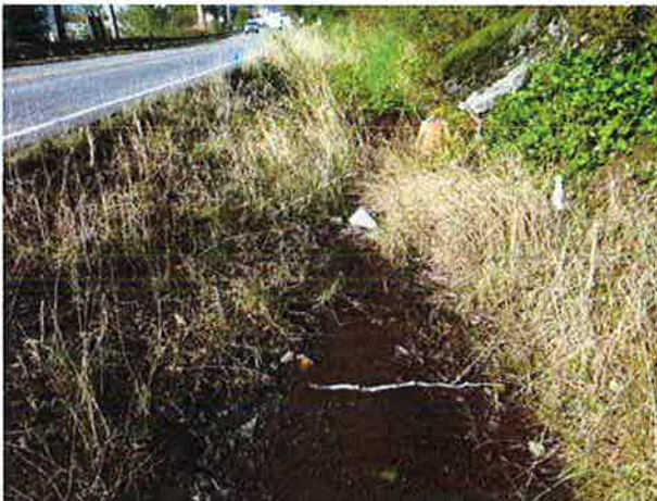
Ditches to north of culvert.
