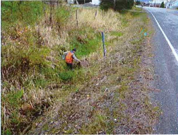
Inlet and ditches to south.
