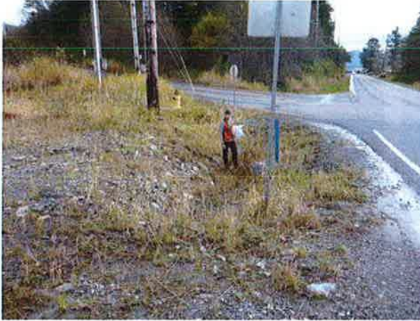
Remove existing culvert, add culvert under spur road, and move water into existing ditch to south (background of photo).
