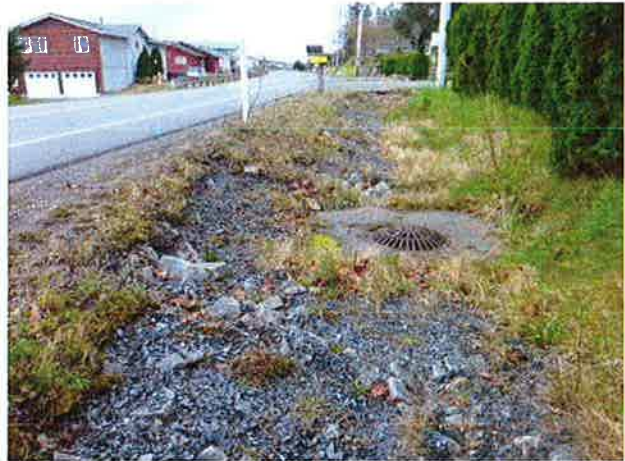
Inlet and ditches to north.
