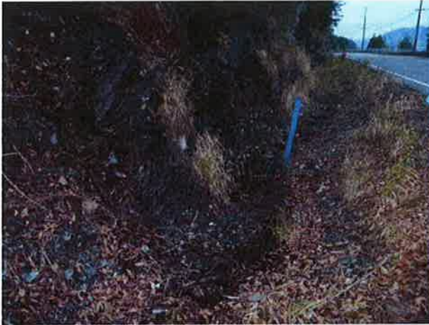
Inlet, rock face, and seep, and ditches to south.
