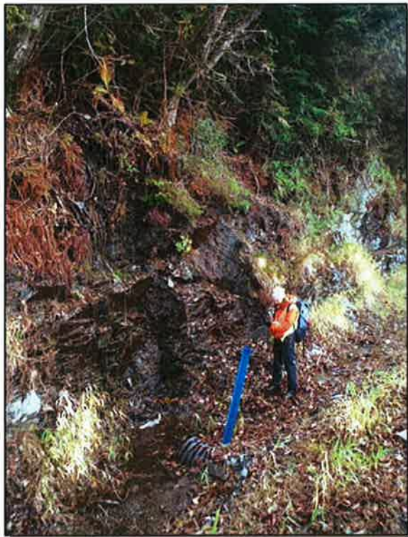
Site 026: Stream Crossing. Photo taken October 15, 2015.
