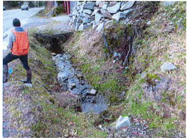
Inlet with driveway culvert, and contribution from property drain to north.
