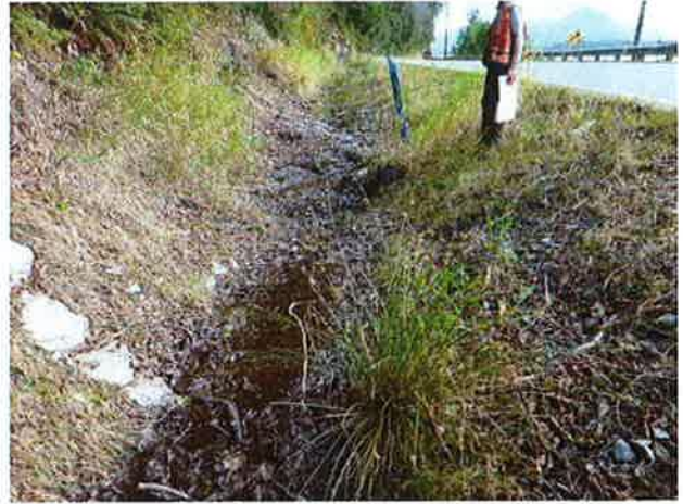
Ditches to south of inlet.
