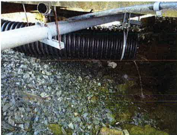
Outlet discharges into ocean. Located under house.
