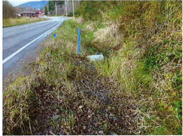
Inlet and ditches to north.
