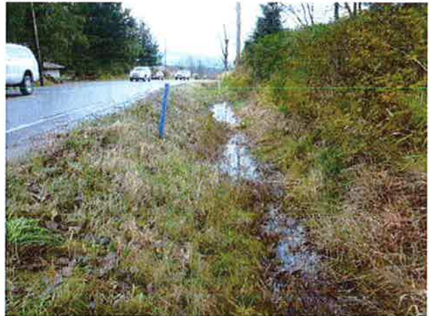
Inlet and ditch to north.
