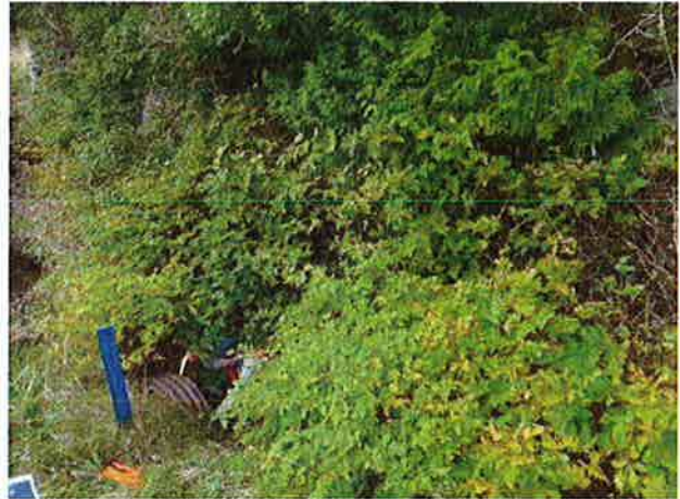
Inlet, view of ditches to north.
