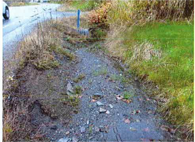
Inlet, ditches, and driveway underdrain to north.
