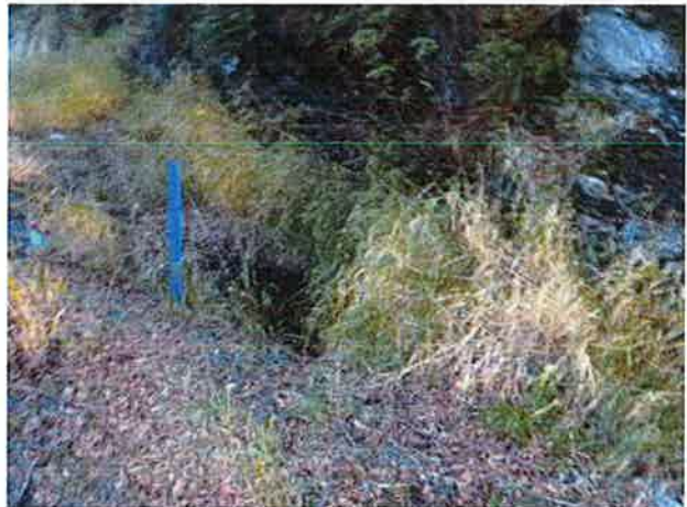
Inlet and ditches to north.
