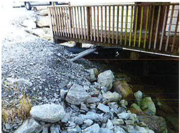
Surrounding structure at outlet. Outlet under deck of house.
