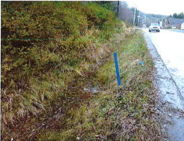
Inlet and ditch to south.
