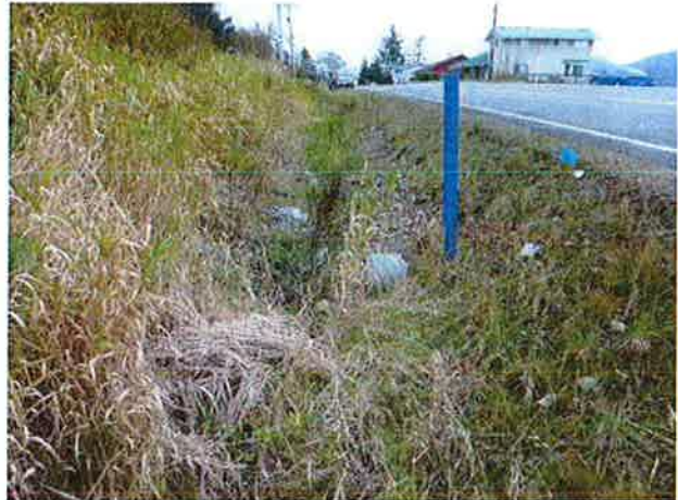
Inlet and ditches to the south.
