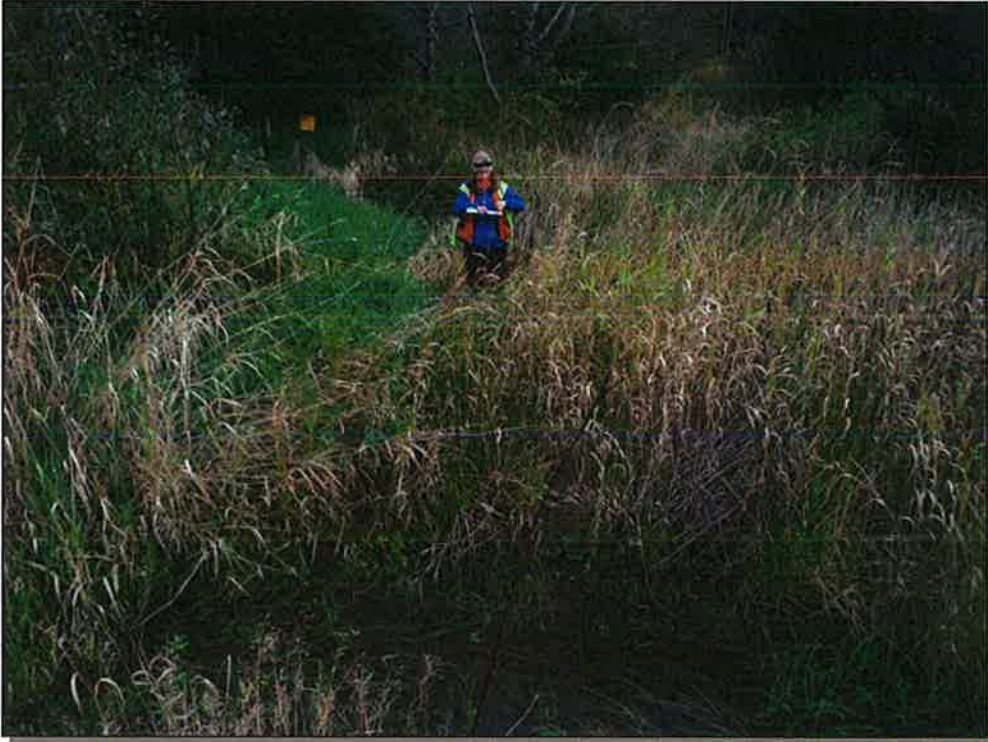
Site 031: Stream Crossing, North View. Photo taken October 15, 2015.
