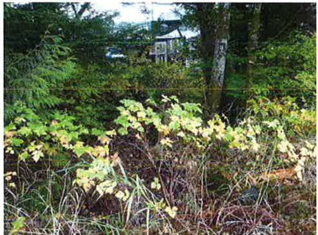
Outlet with no clear ditch or drainage path.
