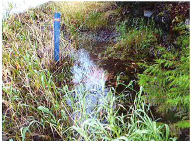
Ponding water at inlet.
