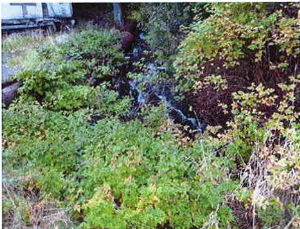
Inlet located below vegetation, stream visible. View from road.
