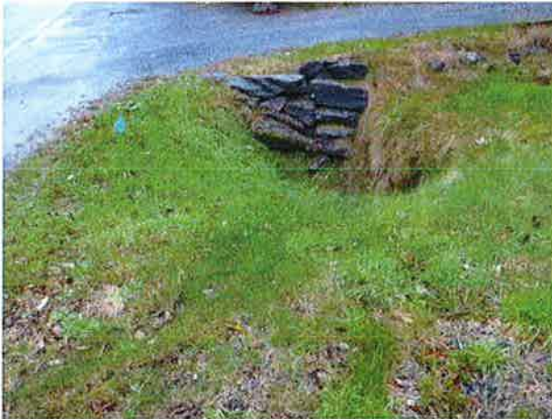
Inlet with driveway to north.
