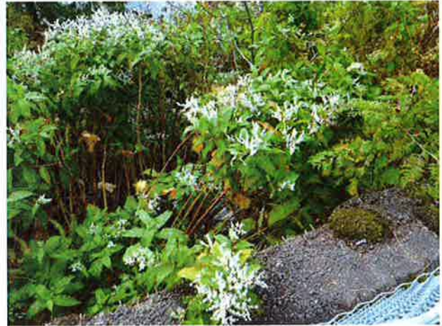
Outlet viewed from above.
