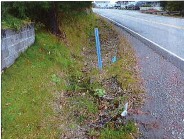
Inlet and ditch to south.
