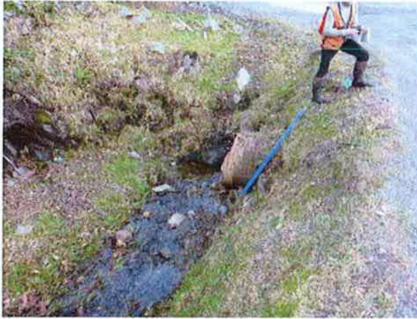
Inlet with driveway to south.
