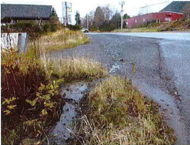
Outlet. Inlet near power pole on far side of road.
