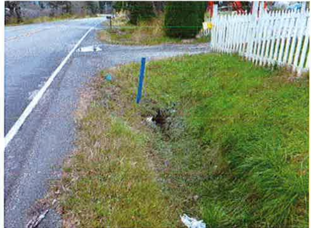
Inlet and ditches to north.
