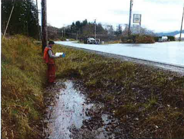
Inlet and ditch to south.
