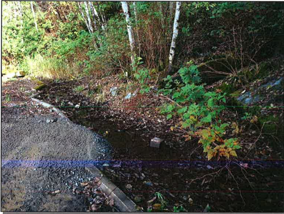
Site 001: Stream Crossing, Upstream View. Photo taken October 14, 2015.
