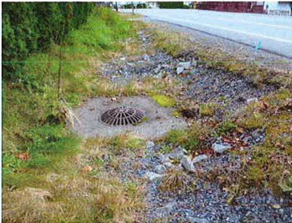
Inlet and ditches to south.
