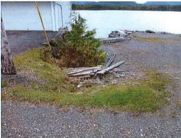
Proposed alignment; culvert with outlet to ditch along vegetated area middle of photo.
