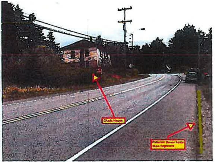
Figure 5. View southeast of the proposed force main alignment in the vicinity of Chief Kashakes House, KET-00343.
