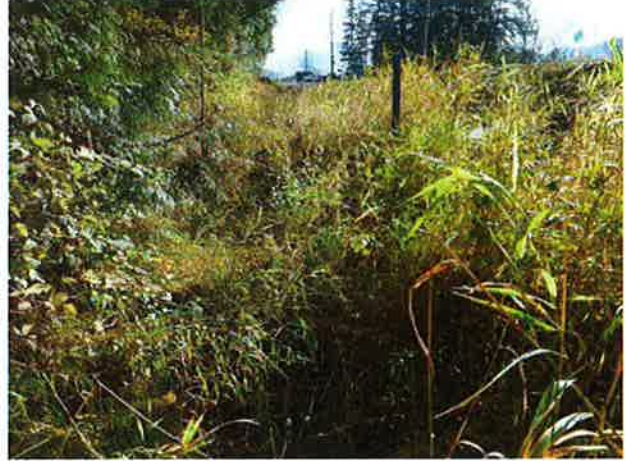
Ditches to south of inlet.
