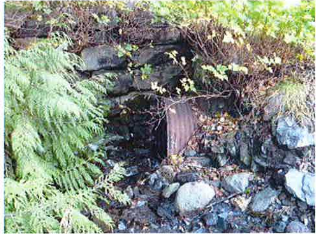
Inlet with rock wall to south.
