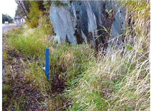
Inlet and ditches to north.
