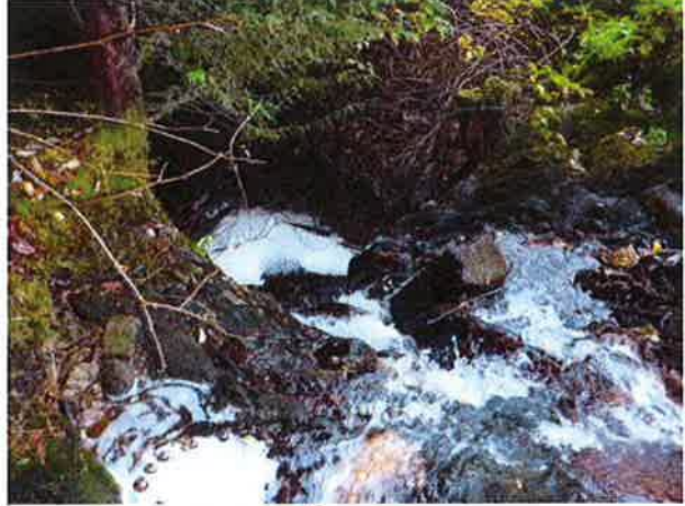
Inlet located at bottom of falls, 15 feet below road surface.
