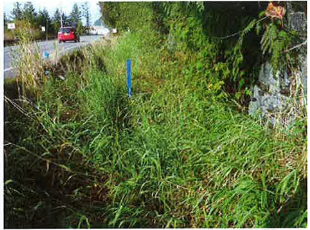
Inlet: Ditch north of culvert. Blue marker indicates inlet location.
