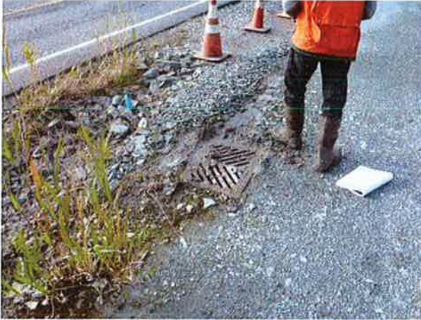
Storm drain inlet.
