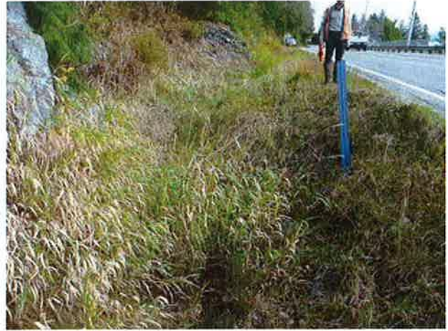
Inlet at blue marker and ditches to south.
