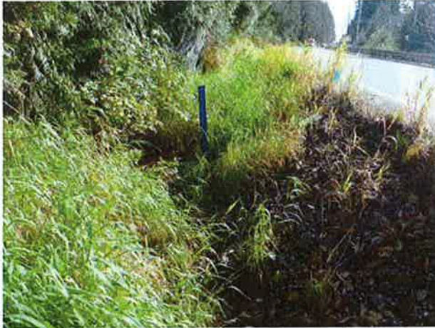
Inlet: Ditch south of culvert inlet. Blue marker indicates inlet location.
