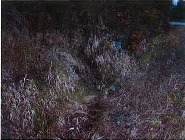
Inlet, seeps, and ditches to south.
