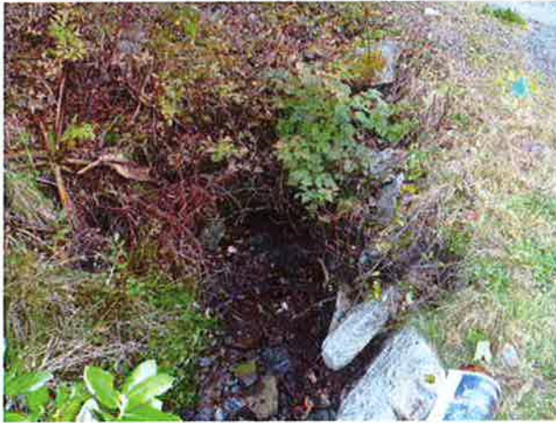
Inlet and driveway to south.
