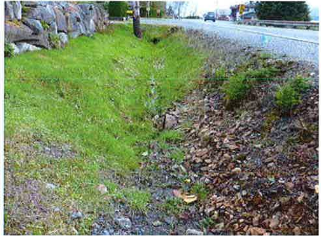
Inlet and ditches to south.
