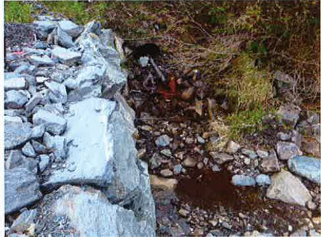
Outlet adjacent to retaining wall.
