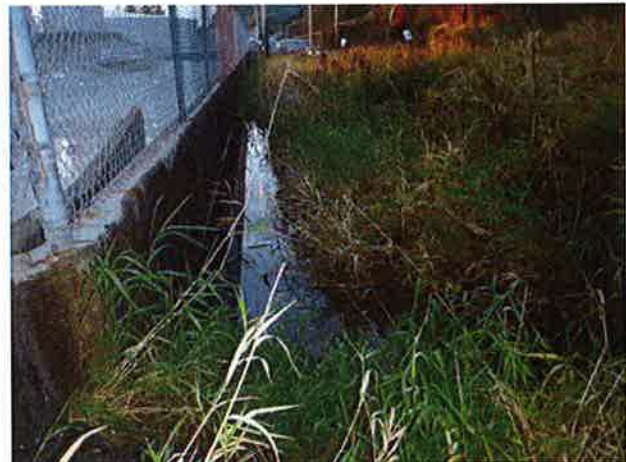
Outlet: Stream flows along concrete barrier wall of fuel tank station.
