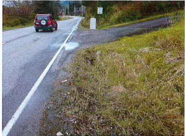
Ditches, driveway, and mailbox near inlet looking north.
