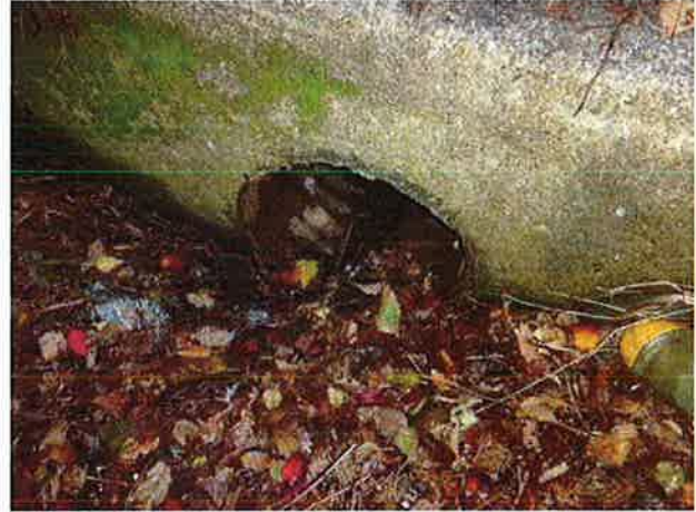
Concrete headwall at inlet.
