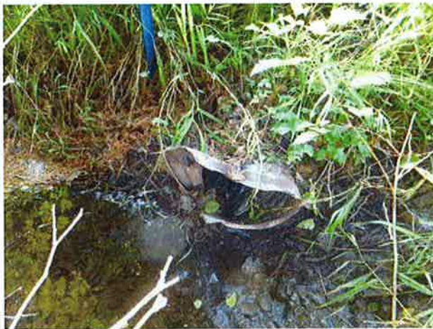
Inlet: Crushed.
