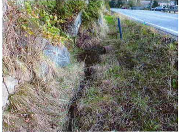
Inlet and ditches to south.
