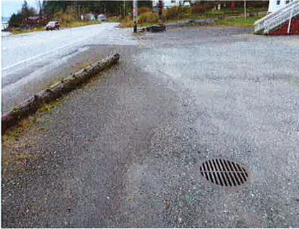
One curb inlet, looking north toward Totem Row Street.
