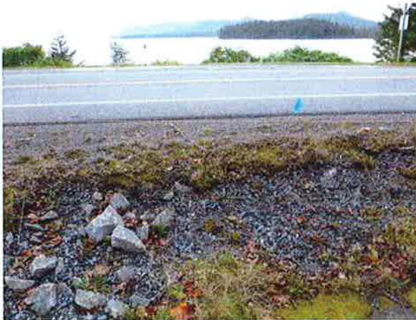
Alignment of culvert under South Tongass Highway.
