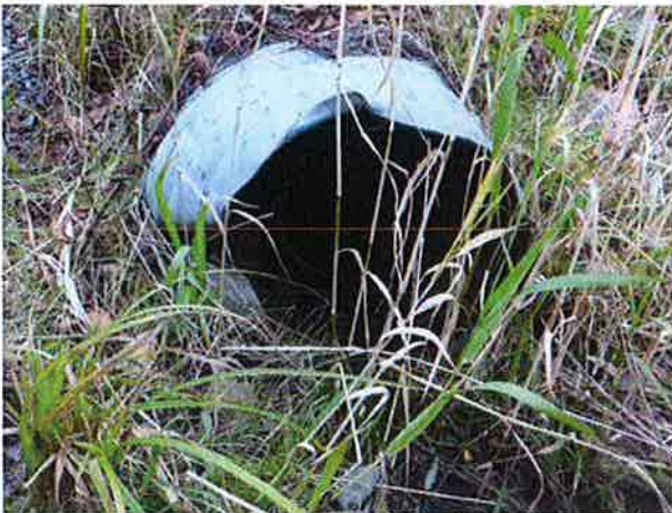
Inlet damaged.
