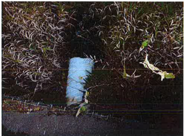
View from top, over fence, of outlet.
