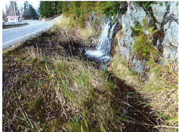
Inlet, falls, and ditches looking north.
