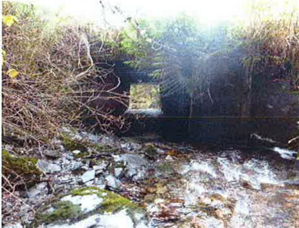
View downstream toward inlet of structure.
