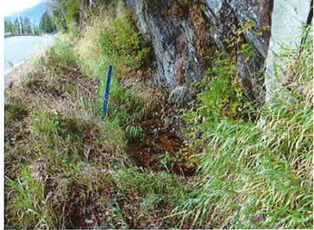
Inlet, rock face, and ditches to north.
